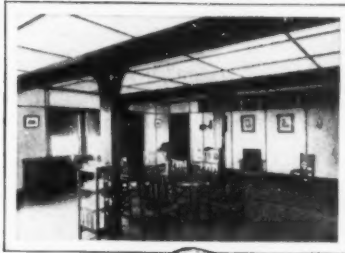
Loosening Room in the Buffalo Motor Boat Club
